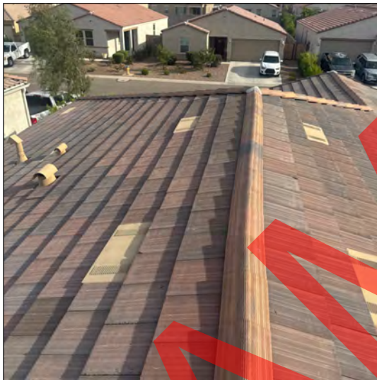
General Roof Surface Photos
